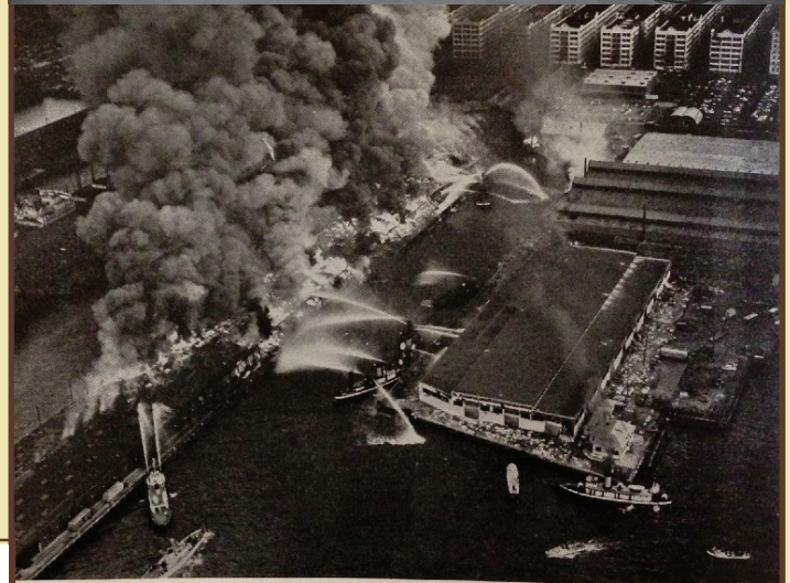
Extent of fire shortly after explosion. Operations of land companies are confined to the shore end while fire in balance of pier must be fought by marine forces. Ineffectiveness of streams from boats where roof has not yet collapsed is very evident. Damage to walls of one story warehouse in right foreground of photo can be seen. Sprinkler piping in this building was broken in many places. U.P. ASSN. PHOTO
