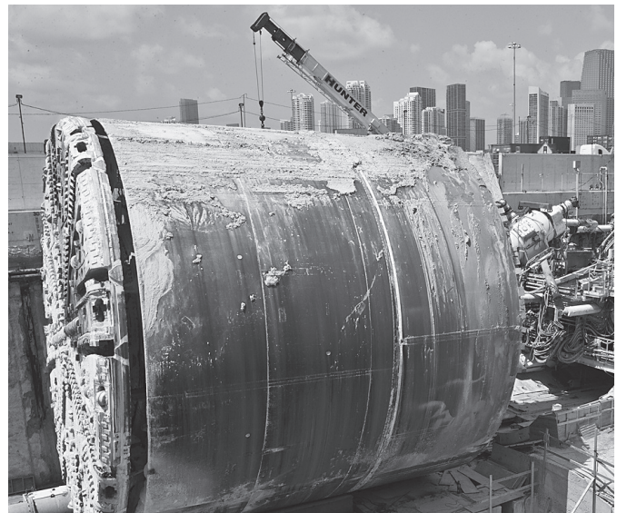
PORT OF MIAMI TUNNEL PROJECT
