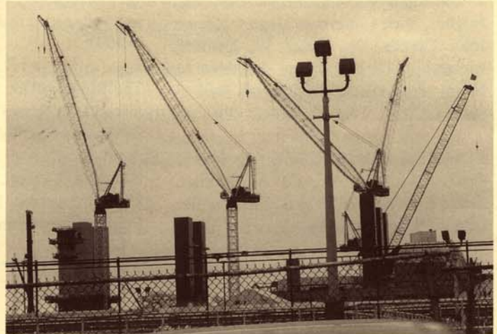
Skyline at Newtown Creek Plant
