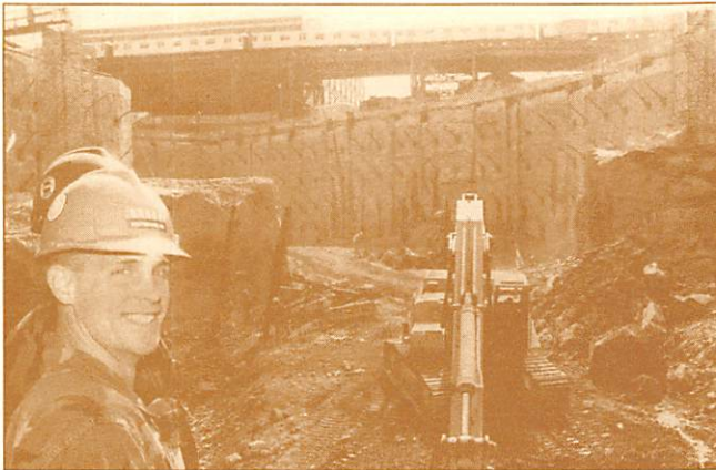
Tied back slurry wall with rock excavation underway.
