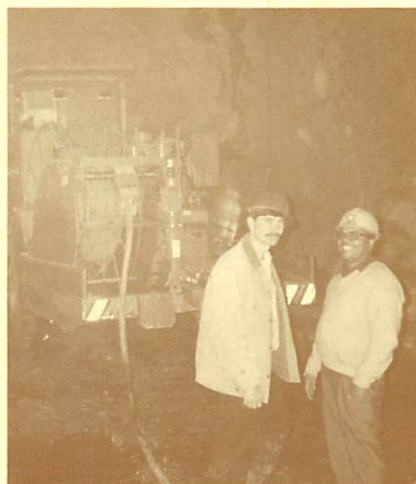
GARY ALMERARIS (left) in Diversion Tunnel Heading
