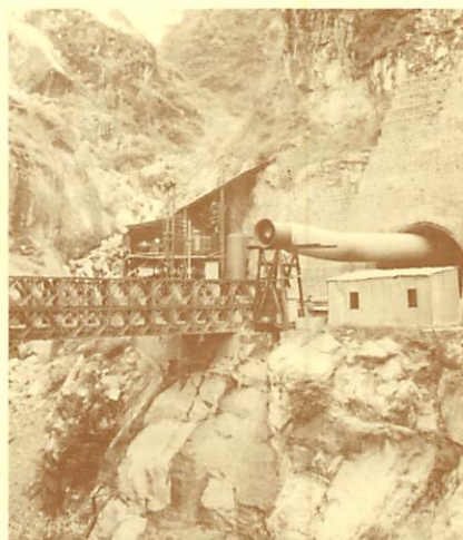
Access to Nathpa Adit Portal
