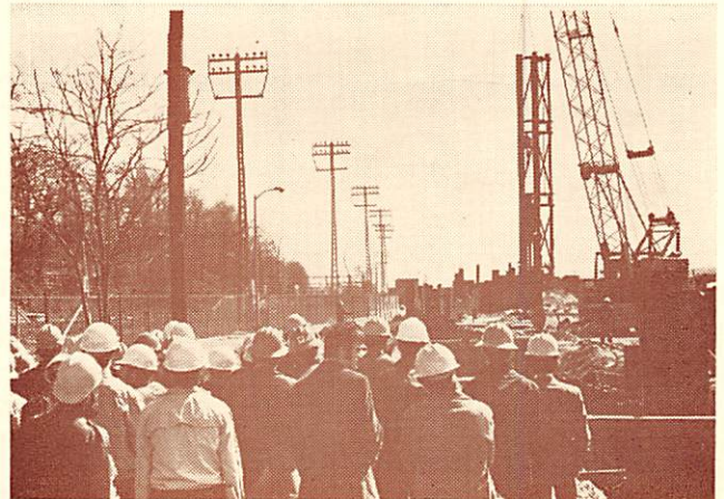
Student Engineers watch pile driving operation at Yonkers Joint Treatment Plant.
