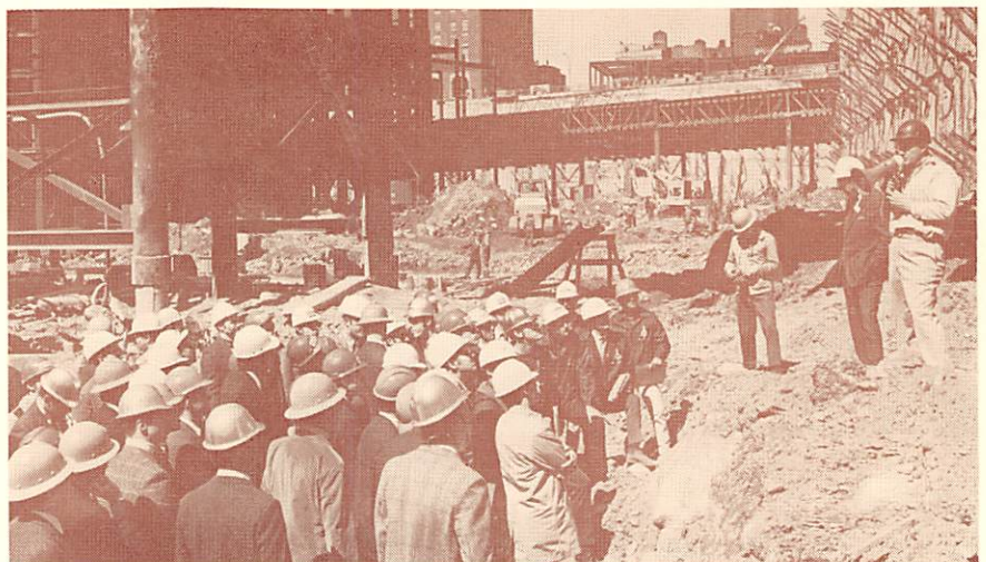
HARRY DRUDING addresses students from south east end of World Trade Center site. View shows slurry wall with tie-backs and trestle for PATH Tube in background.
