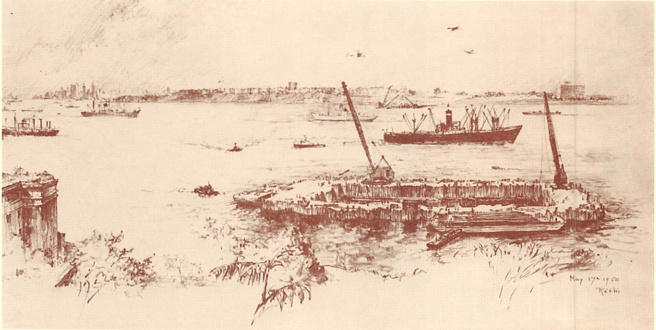
GENERAL VIEW OF EARLY CONSTRUCTION of Verrazzano ("Narrows") Bridge across New York Harbor, looking from Staten Island across to Brooklyn.
